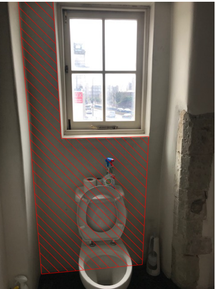
Part of Bromley Hall to be Removed to create Doorway
